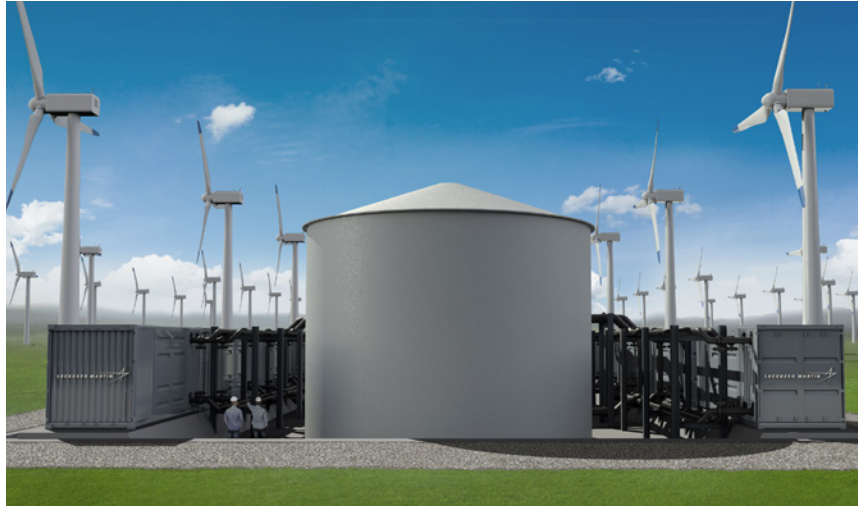
Figure 4: Rendering of 10 MW x 10 hr GridStar® Flow System at a wind farm
